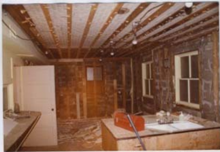
26 April 1983 started work on the kitchen. Baptismal Font removed.
