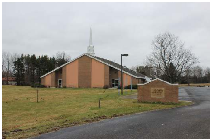
Current Phase 2 Building on 72 nd Avenue in Hart
